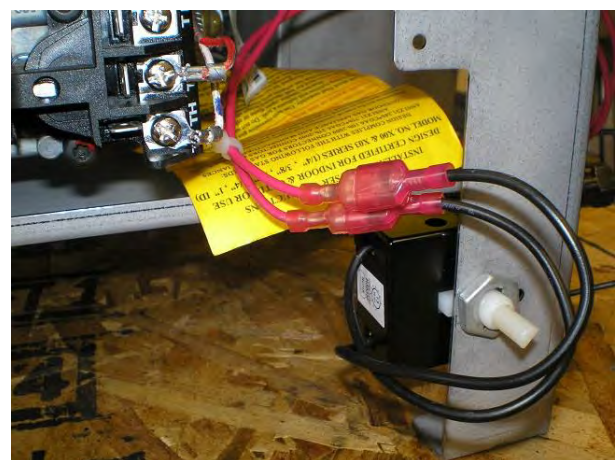
5. Connect wiring.
