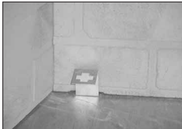
Figure 8.8 Grate Retaining Bracket in Place
