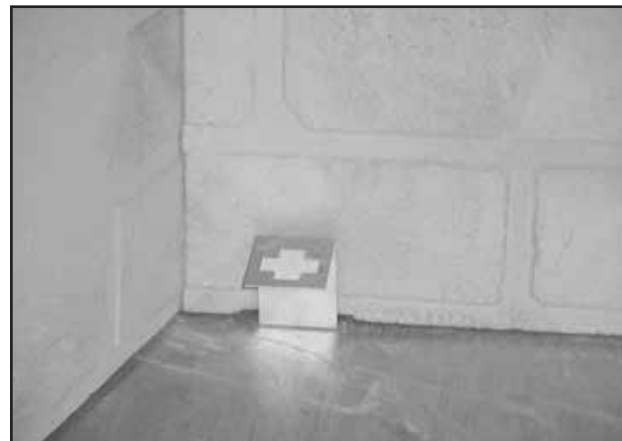
Figure 8.8 Grate Retaining Bracket in Place
