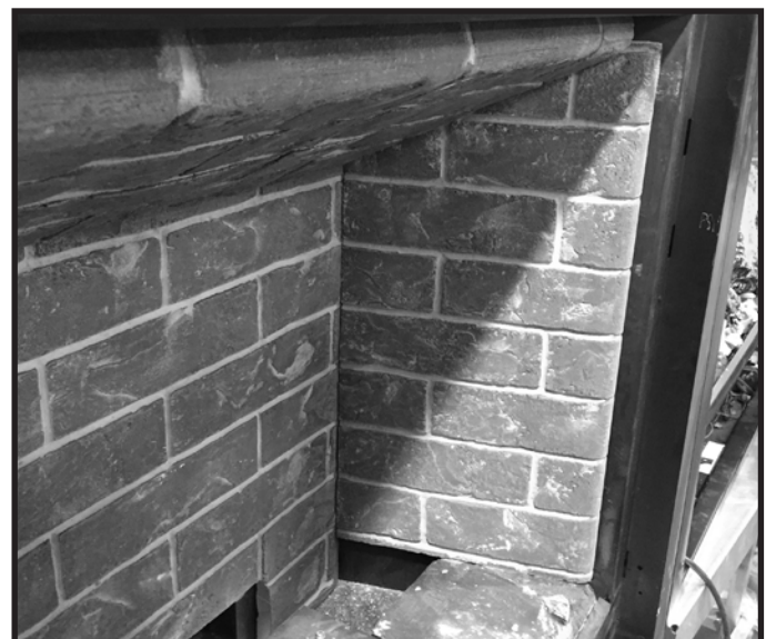
Figure 11.6 Right Refractory Panel Installed
