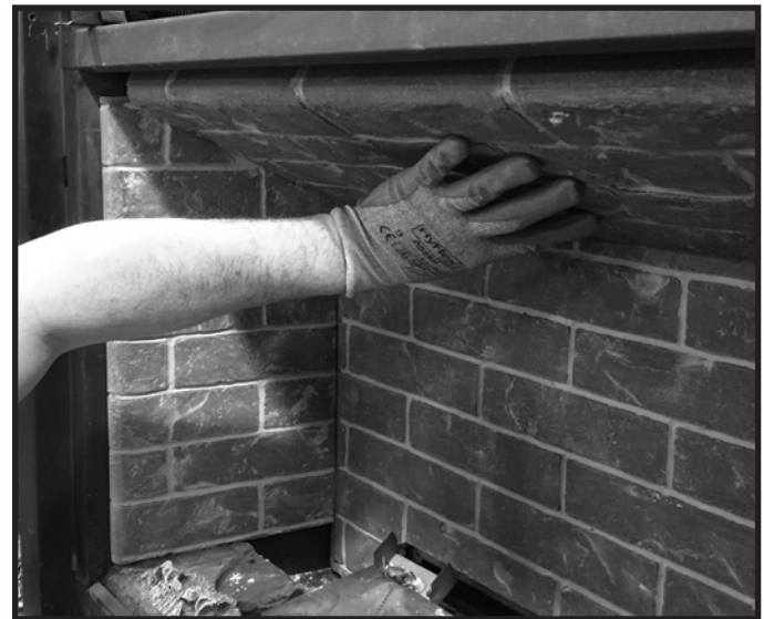
Figure 11.5 Install Right Refractory Panel
