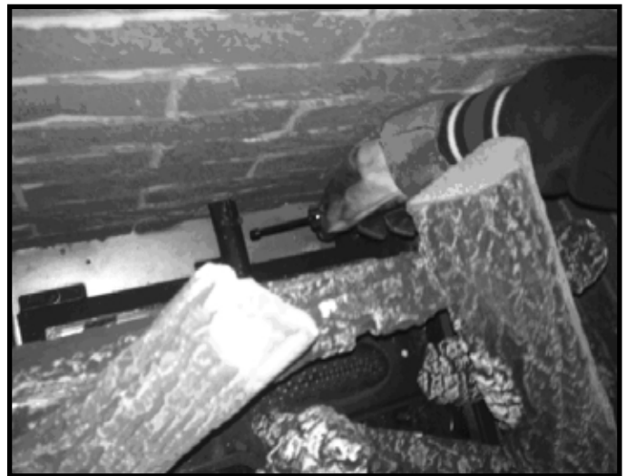
Figure 9.1. Air Shutter Location
