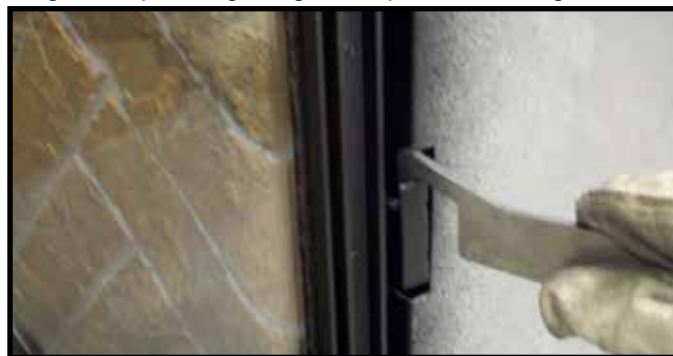
Figure 11.7. Securing Side Glass Clips
