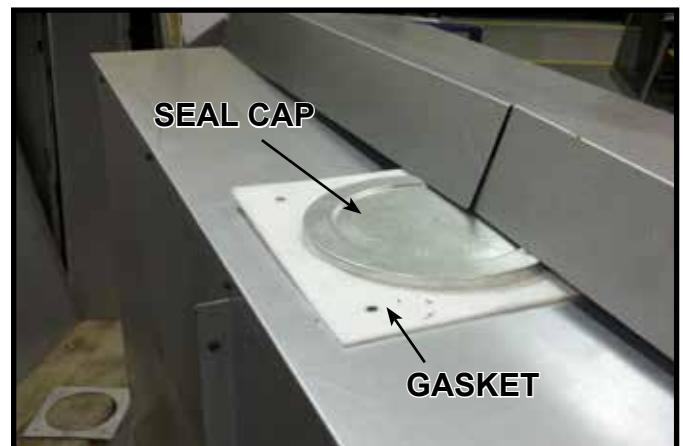
Figure 6.2 Seal Cap and Gasket Location
