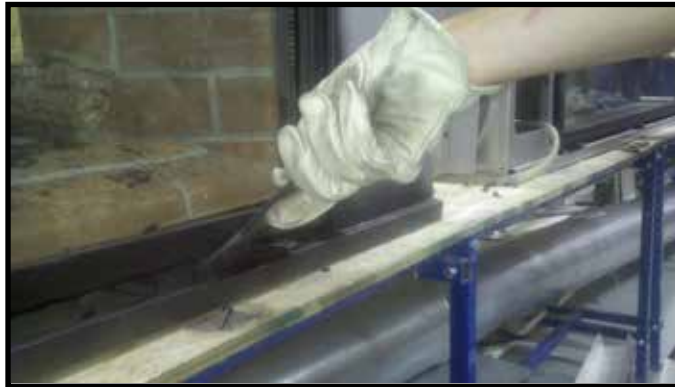
Figure 11.3. Inserting Glass Clip Tool
