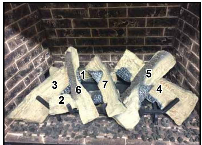
Figure 17. Log Set Installed.
