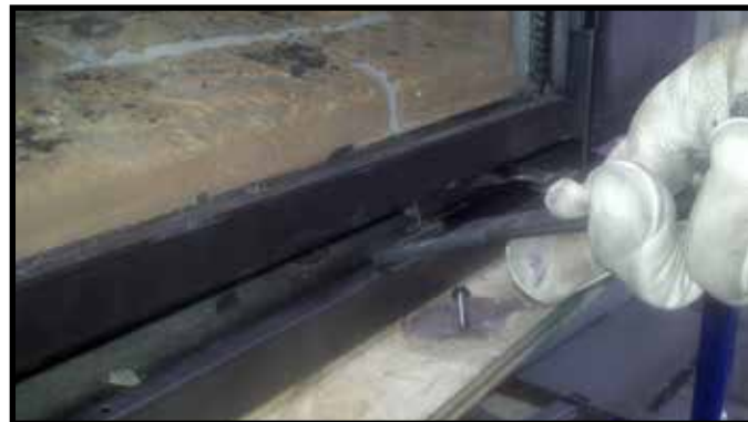
Figure 11.2. Glass Clip Tool Location
