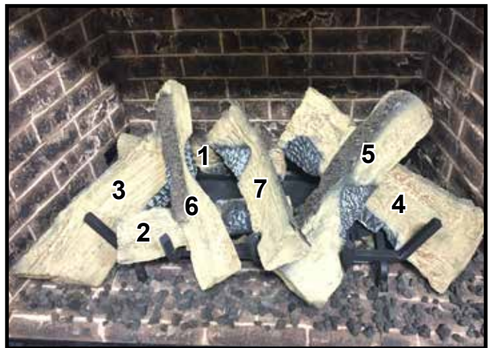
Figure 16. Log Set Installed
