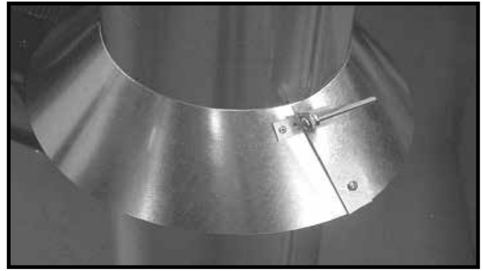
Figure 7.12 Insert Bolt into Brackets
