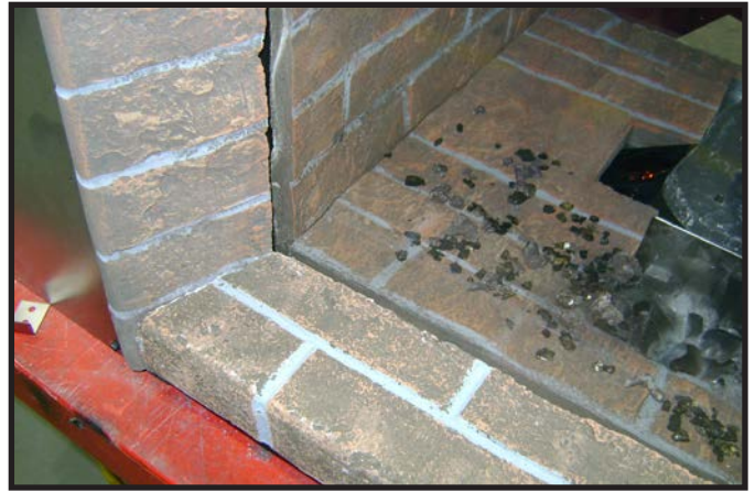
Figure 11.28 Outer Hearth Installation
