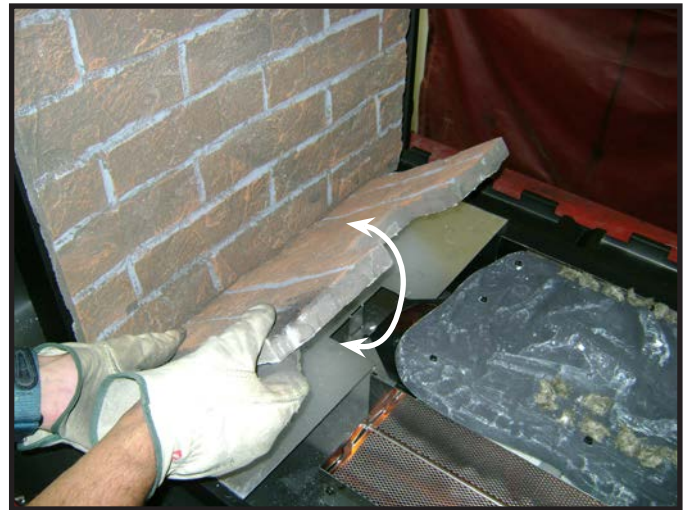
Figure 11.17 Positioning Inner Bottom Refractory
