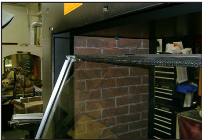
Figure 11.2 Initial Positioning of Frame into Opening.
