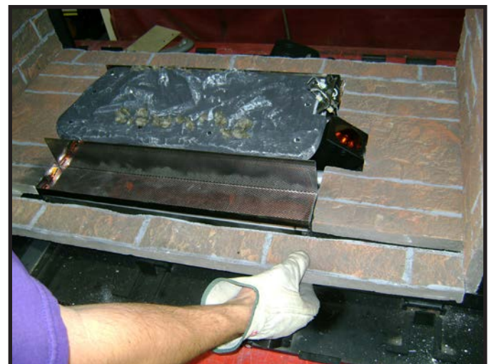
Figure 11.19 Positioning Outer Bottom Refractory.
