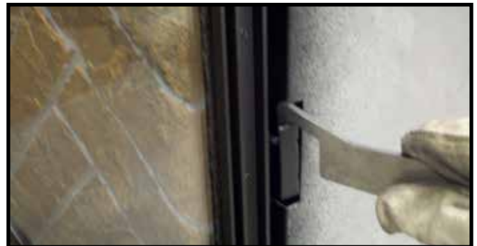
Figure 11.7. Securing Side Glass Clips
