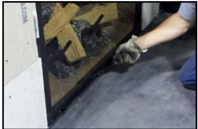
Figure 11.8. Securing Bottom Glass Clips
