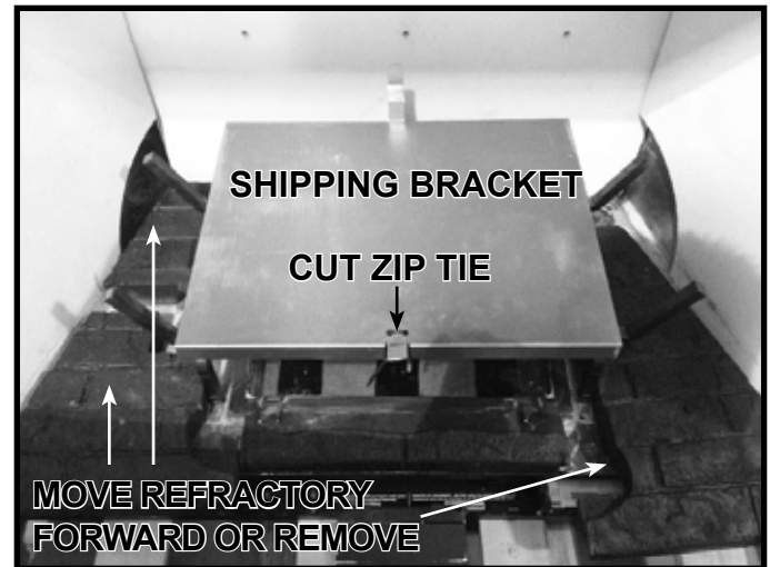
Figure 11.10 Separate Shipping Bracket from Log Grate
