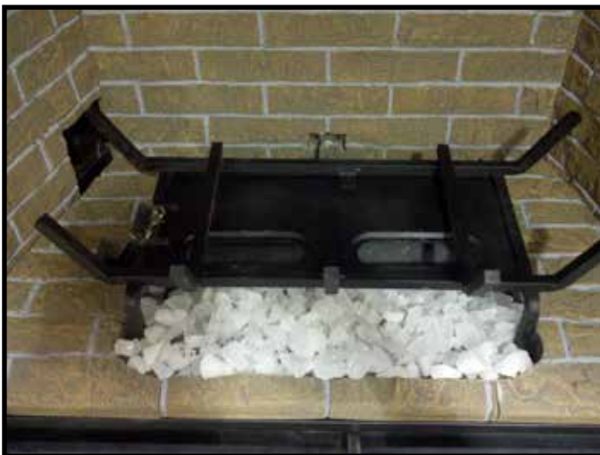
Figure 11.20. Ember Glass Area Covered with Teco-Sil
