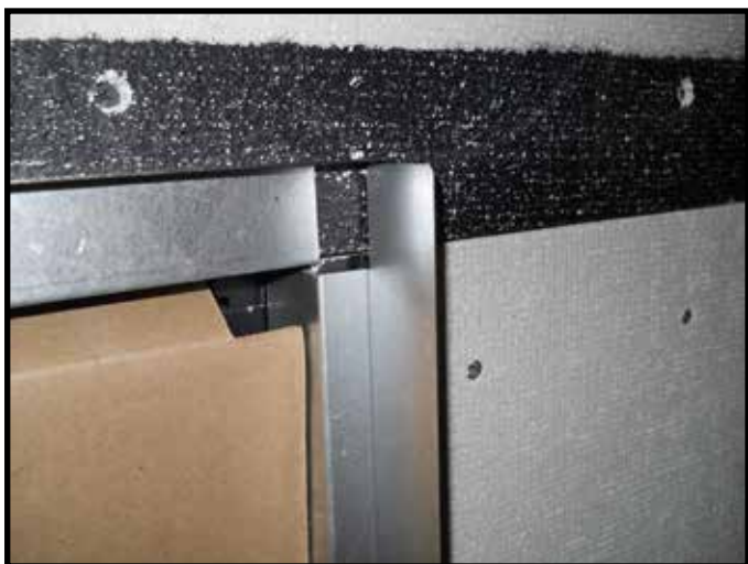
Figure 10.5 Finishing Template Bends
