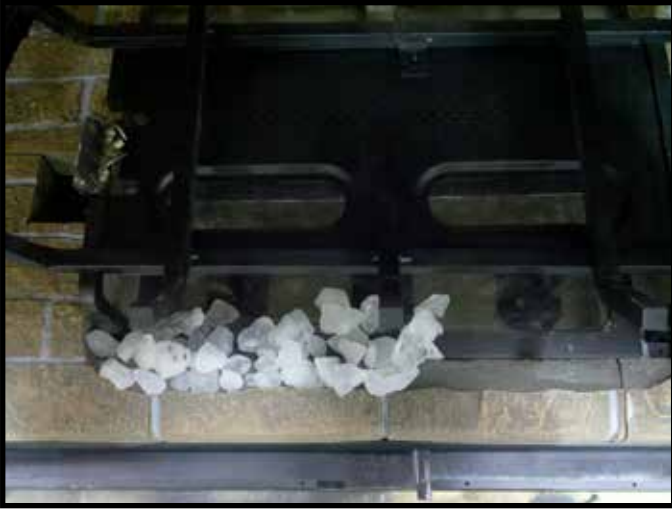
Figure 11.19. Install Teco-Sil
