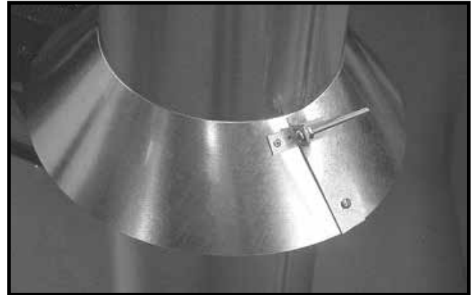
Figure 7.12 Insert Bolt into Brackets
