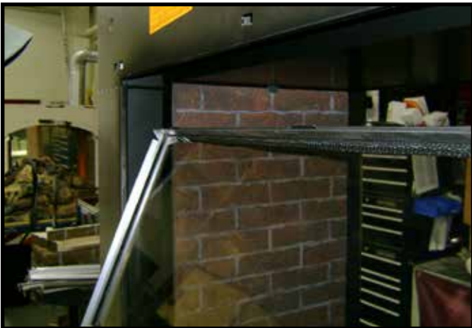
Figure 11.2 Initial Positioning of Frame into Opening.
